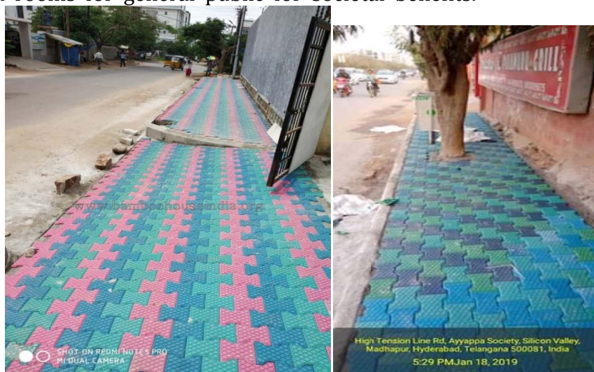
Tiles from Waste Plastic installed by Municipal Corporation, Hyderabad
