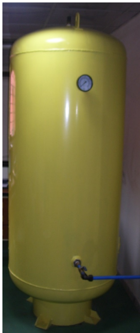
(b) Air Receiver of 1000 L Capacity
